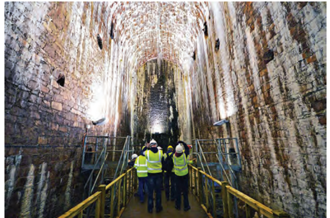
Inside the transverse chamber (the second one visited) looking east, showing the scale of the vault, the numerous straw stalactites, and side platforms leading to crawl holes though to the outer chambers
